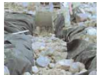
Filling the toe
