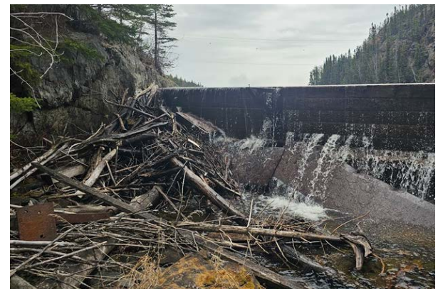
Top: Before clean up Bottom: After clean up
