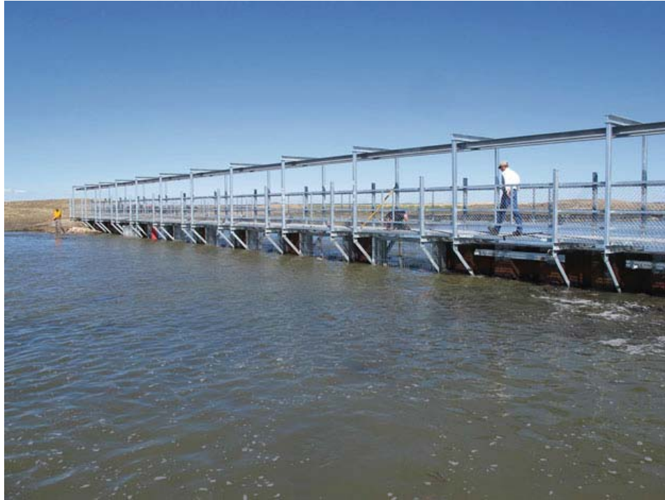
Fig. 9 In early 2013, seven structures were constructed to exclude most large common carp from Delta Marsh as a means of restoring submersed macrophytes and other components of the coastal wetland ecosystem degraded by this invasive, benthivorous fish (Photo credit: D. Wrubleski © Rights remain with the author)
