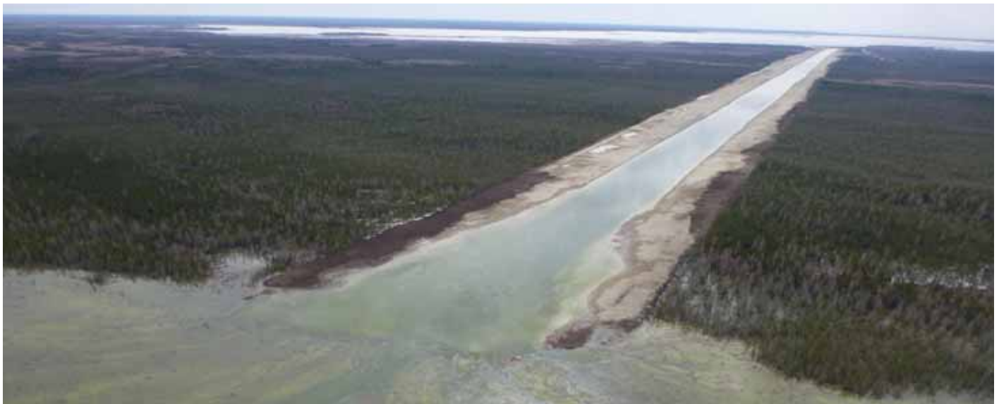
Lake St. Martin Emergency Outlet
