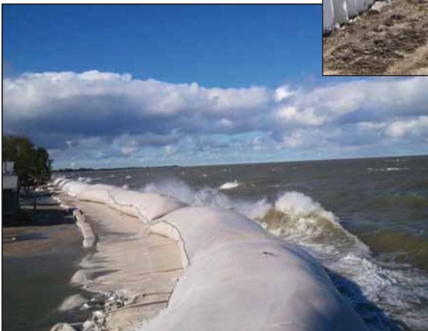
Flood Tubes at Lake Manitoba Basin
